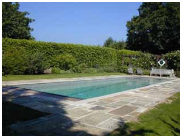
Sawn York Copings with Re-claimed York Paving
