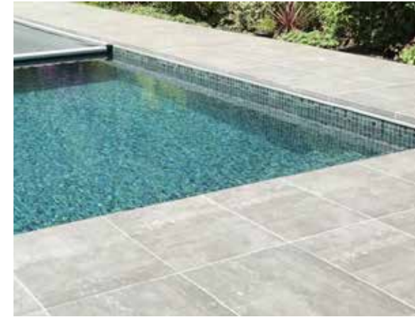
Porcelain Over-lip coping with automatic pool cover system
